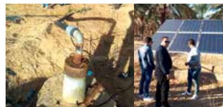
*Solar pumping system using the new SIPS product.*
