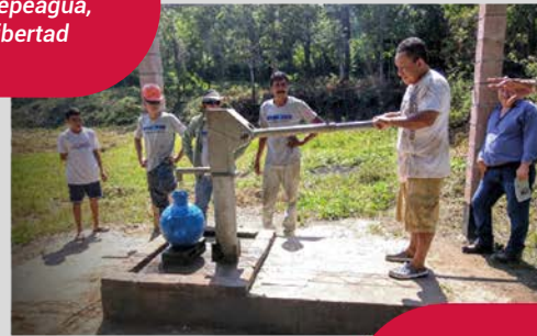
Drilling and pump for well on Ca/Valle Nuevo, Victoria, Cabañas
