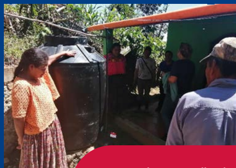
Rainwater collection system in Aldea Chilley, San Cristóbal, Alta Verapaz
